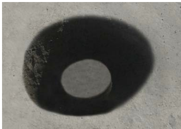
Fig.2 DEHA/Kontakt SK transportankare
